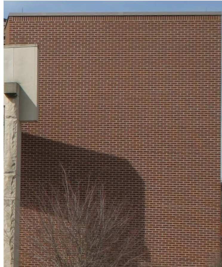
Properly sampled image of brick wall
